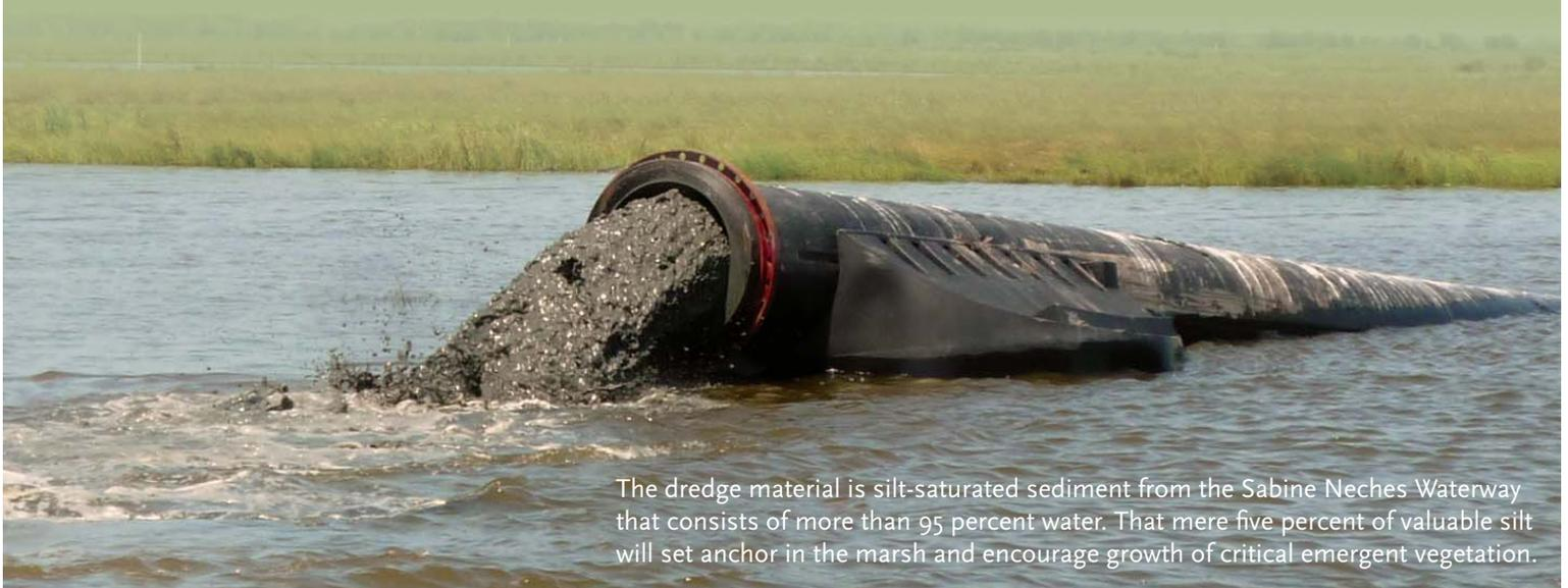
The dredge material is silt-saturated sediment from the Sabine Neches Waterway that consists of more than 95 percent water. That mere five percent of valuable silt will set anchor in the marsh and encourage growth of critical emergent vegetation.
