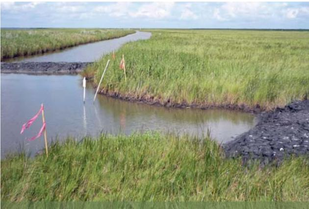
Ditch plugs were constructed where existing access channels and tidal sloughs from Keith Lake join the project's fill areas. These plugs will contain the dredged material, force the sediment-laden dredge water to flow into the existing vegetated marsh plain, and allow for de-watering.
