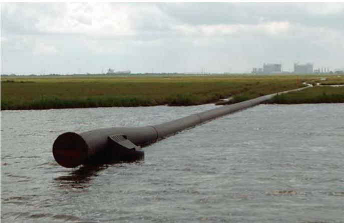
Dredge materials were piped more than 4 miles from the Golden Pass LNG berthing facility through a temporary pipeline.
